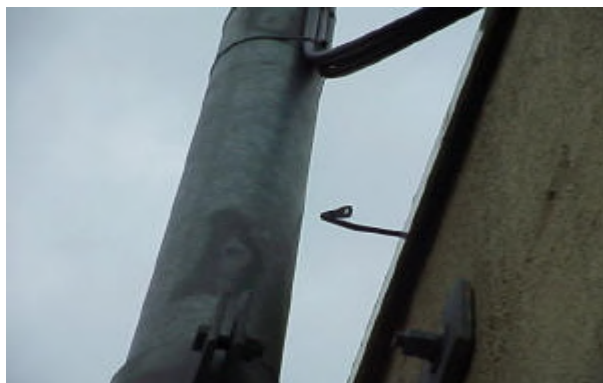
Losse verbinding
